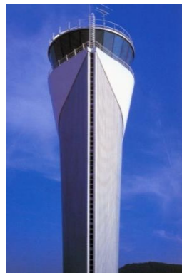
Sondica Airport Tower
